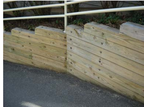
Retaining wall good condition
