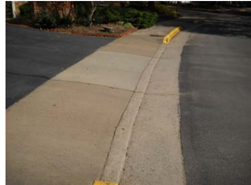
Sidewalk, apron, gutter
